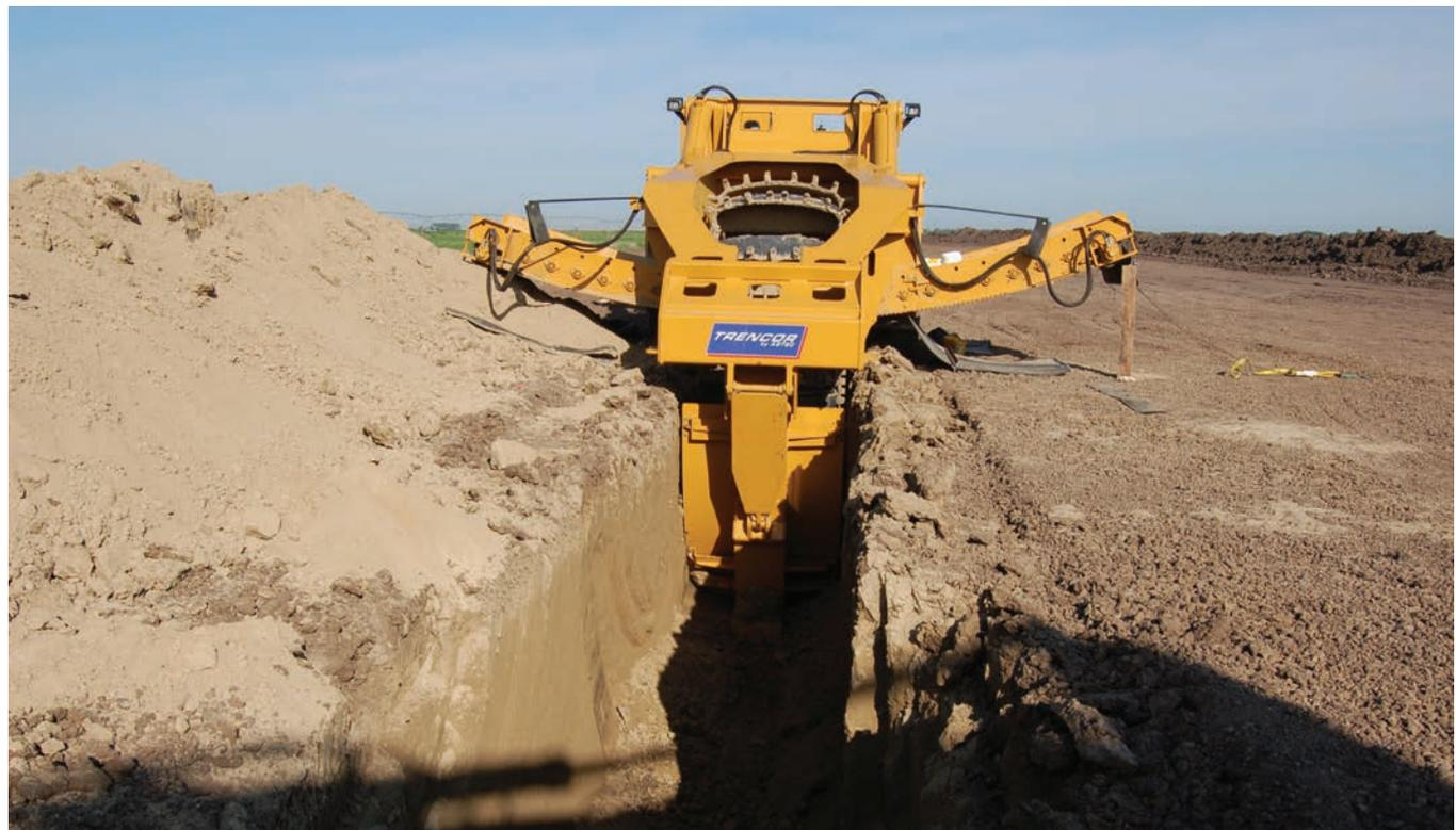
**DIGGING ACROSS NEBRASKA:** A trencher does its work during construction of the first Keystone pipeline in Nebraska a couple of years ago.
